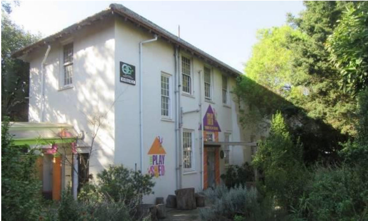
Photograph 4.21: Entrance to The Play Shed, Block G.
