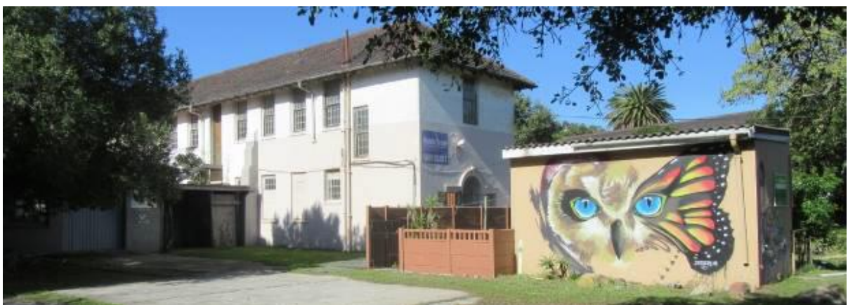
Photograph 4.8: Robin Trust’s Homebased Carer College, front (western) portion of Block F
