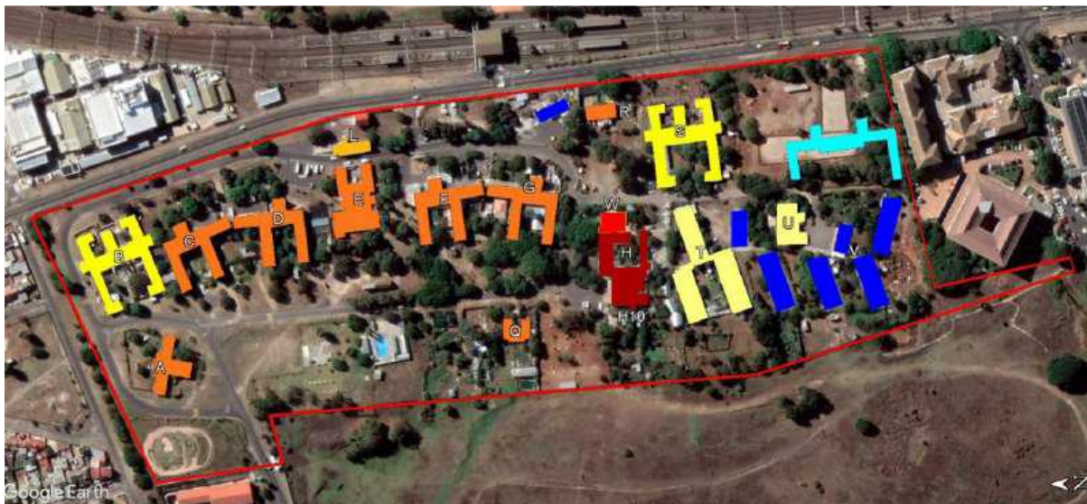
Figure 34: Valkenberg East Hospital on the OMP site at its greatest extent, around 1977. Note the block referents A to V are indicated and referred to in the text. Construction dates of main buildings on OMP site: 18th Century homestead core and later extensions (dark red fill), 1900c (red), 1917-1920 (dark orange), 1920-30 (light orange), 1957-1966 (dark yellow), 1973-77 (light yellow). The large C-shaped old hospital building was constructed 1917-20, and demolished sometime after 1988 (light blue). Prefabricated buildings constructed 1973-77 and demolished during the 1990s in dark blue fill. Apart from the farmstead complex, all existing main buildings on the site date to the Valkenberg Hospital period (Source: O'Donoghue).
