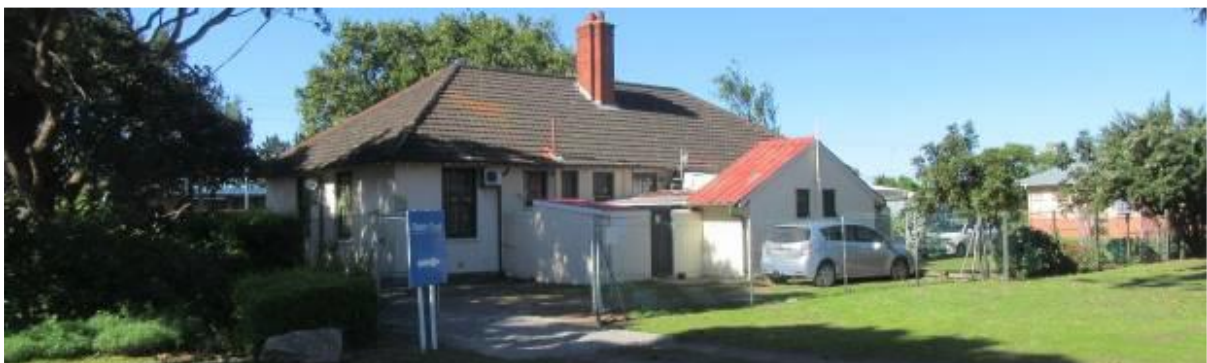
Photograph 4.7: Robin Trust, administrative building (Block R).
