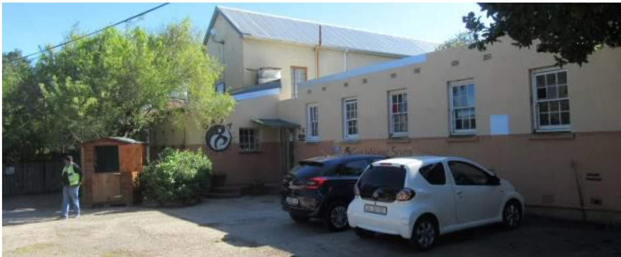
Photograph 4.3: South entrance to the Gaia Waldorf School's original premises, Block H
