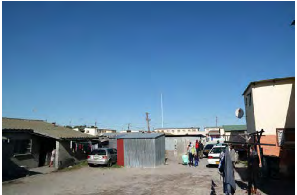
View of some structures in Hlazo Village
