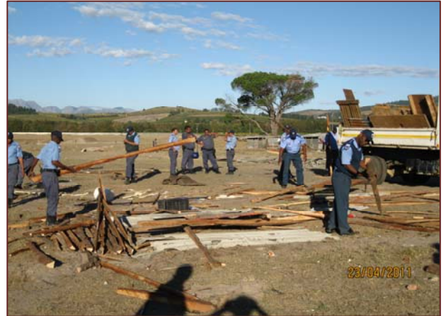
Figure 8: Demolishing of illegal structures
