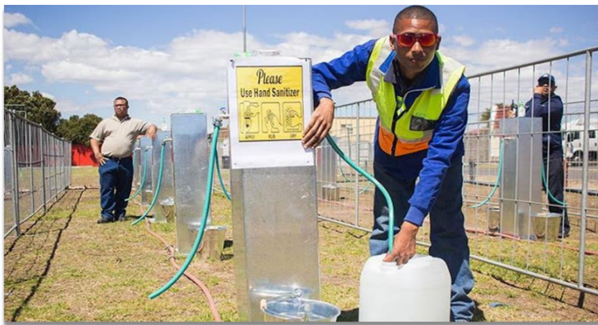
Figure 2: Trial demonstration of one of the water supply Points of Distribution that would need to be established across the city for all residences to receive their water allocations if Day Zero was reached.
