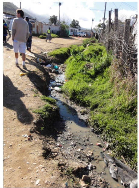
Plastics and solid litter collect in gullies formed by polluted grey water and stormwater which run downhill through the middle of the settlement.
