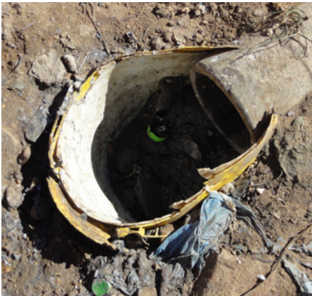
Residents dispose of grey water into these buckets which then flows into the existing underground pipe system they have installed. The existing network functions inadequately but will be used as a foundation for the new network of “living sewers”.
