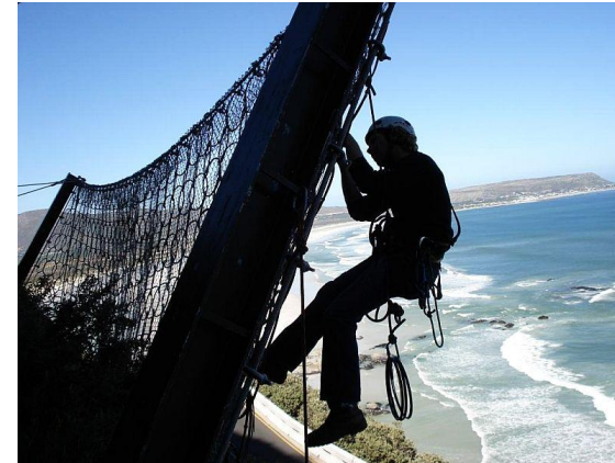
Rehab: Climber Inspecting a Catch Fence
