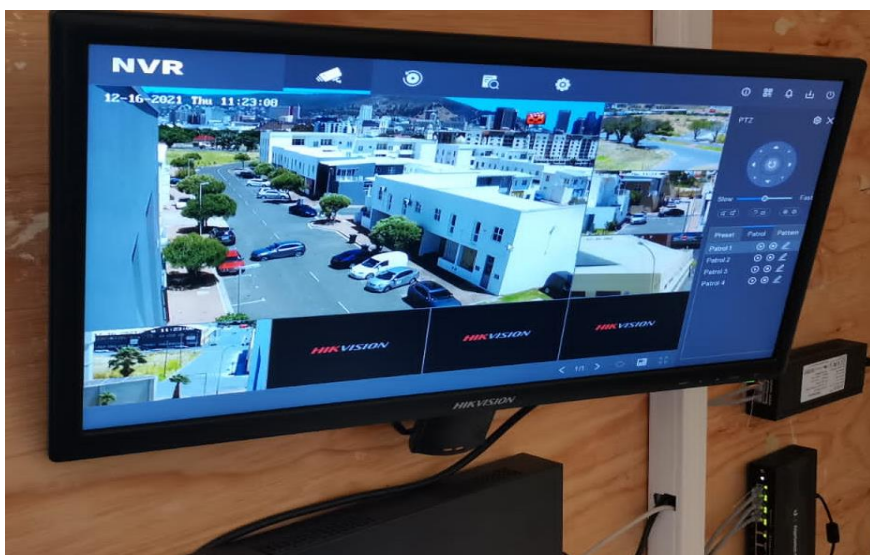
▲ The view of the CCTV cameras in District Six.
