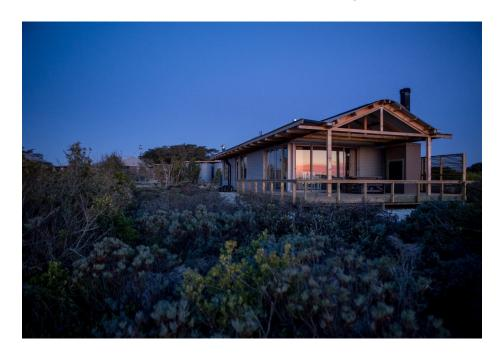
Rocherpan Nature Reserve up the cape's West Coast is home to eight lightweight eco-cabins featuring roofs that harvest rainwater; lightweight construction with minimal foundations; passive cooling design; waterless composting toilets and a recently retrofitted photovoltaic energy supply ensuring a robust off-grid approach.
