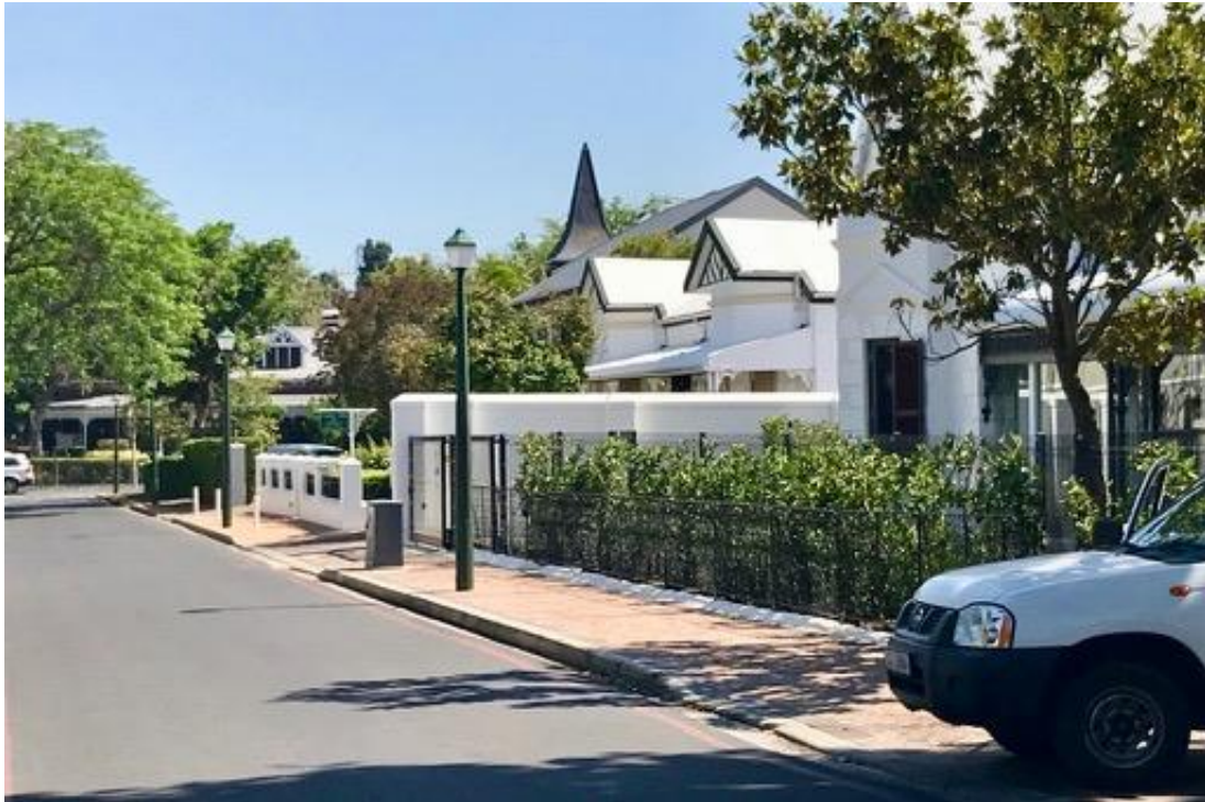
FIGURE 03: The Neethling St streetscape looking north towards Van Riebeeck St. The subject site is in the foreground, right.
