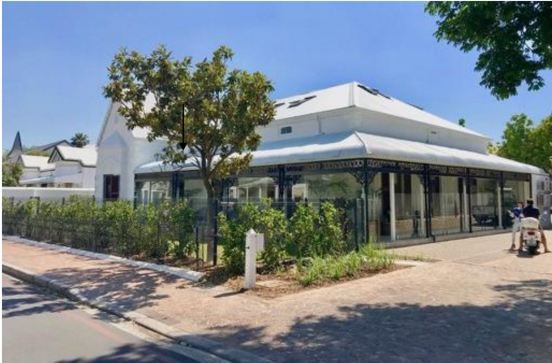
FIGURE 01: View of the subject property from Neethling Street.
