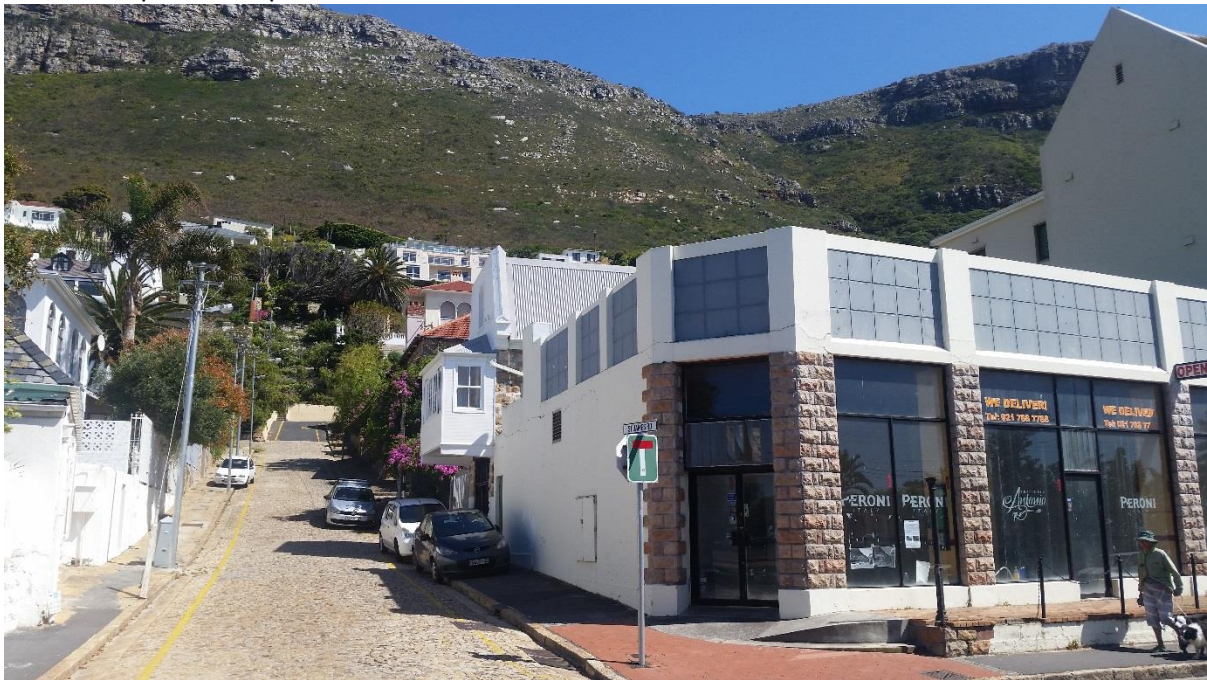
Figure 1 56 Main Road, St James
