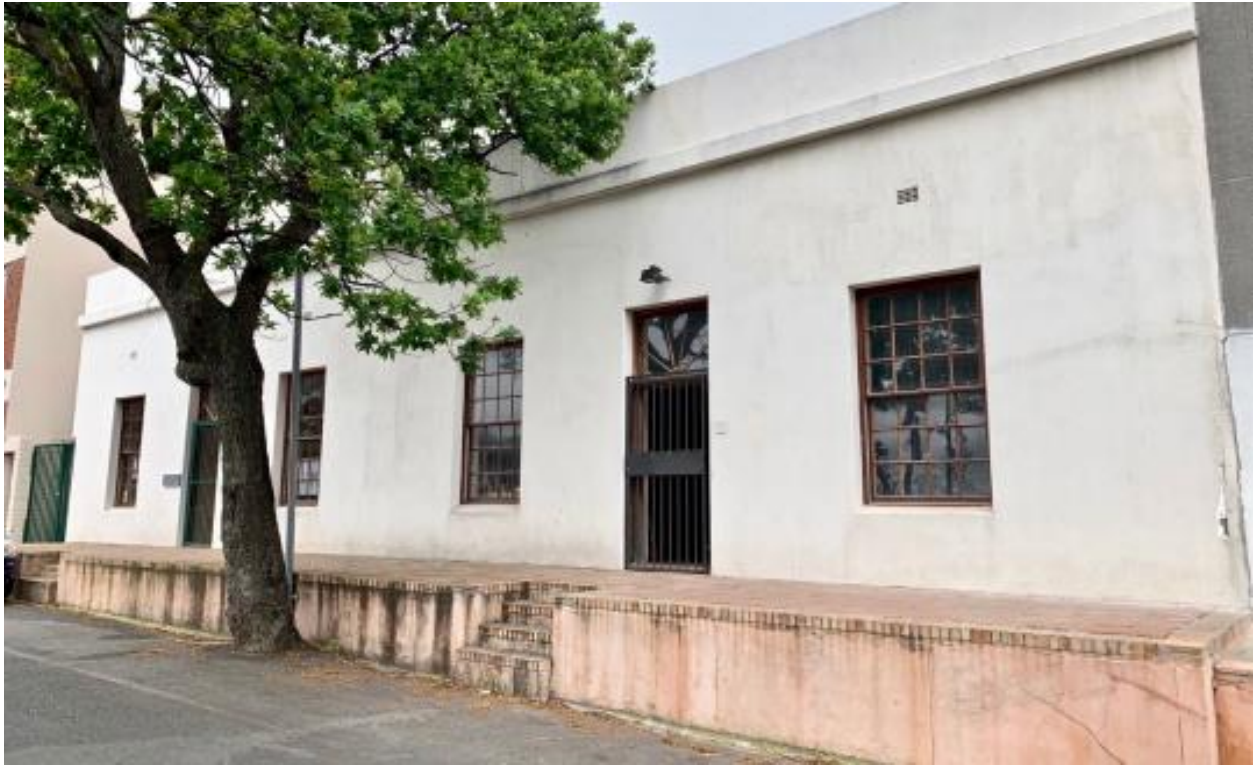
FIGURE 01: The plain front façade of the subject site.
