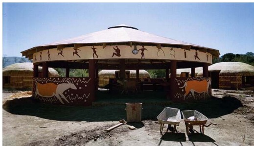
A Shelter Under Construction At Khoi-San Village in the Northern Cape
